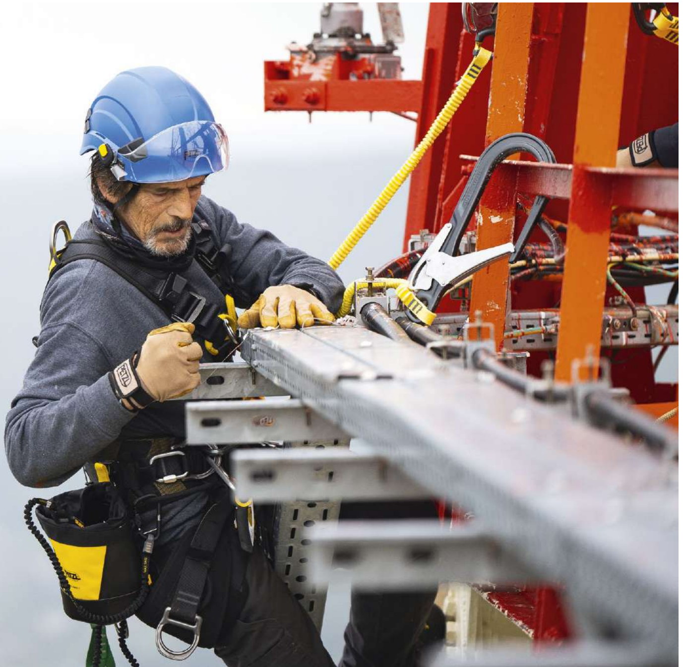
Maintenance operations on a communication tower, Belgium © 2023 Petzl Distribution - Vuedici.org - Monnaie
