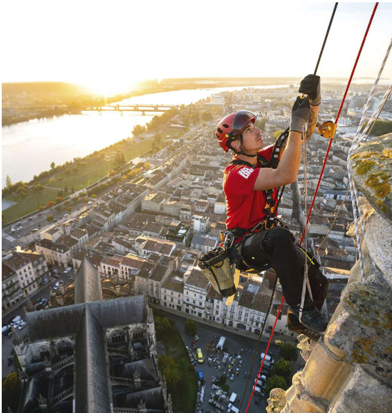
Installing monitors on the spire of the St Michel Church, Bordeaux, France © 2021 Petzl Distribution - Vuedici.org - Adrenaline - Bordeaux City Hall
